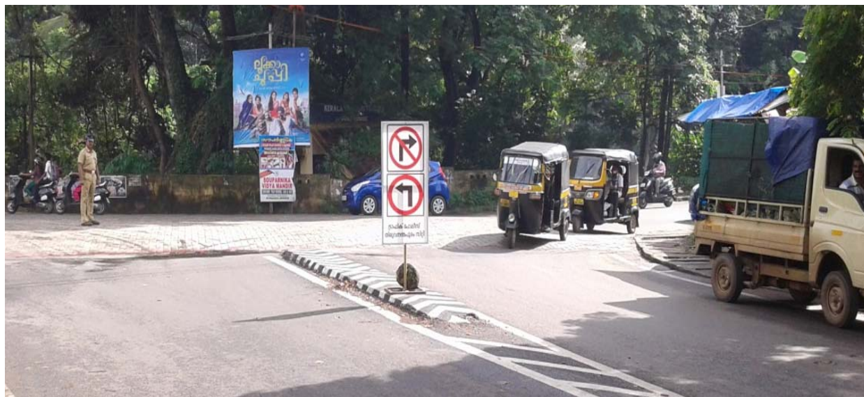
Plate 10: 'No right turn' board installed as recommended by NATPAC
