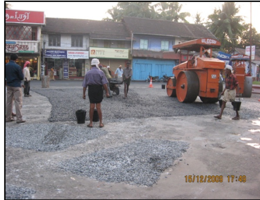
Plate 5 Resurfacing using Modified Mix with PCA
