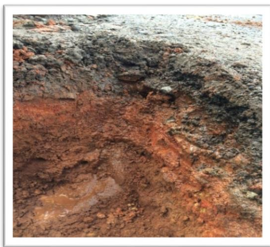
Plate 3: Seepage of water in base course
